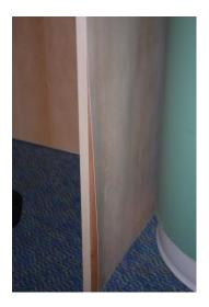
Veneer separated from end panel of circulation desk. Staff noticed that the veneer was separating from a panel of the circulation desk. Schiavone Construction was contacted and, withing a matter days, repaired the panel. An inspection of the desk did not reveal any other problems.
